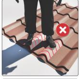
STEPPING ON THE ASSEMBLED METAL ROOF IS ALLOWED ONLY ON THE AREAS BETWEEN THE CORRUGATED PARTS OF THE METAL PANEL.
